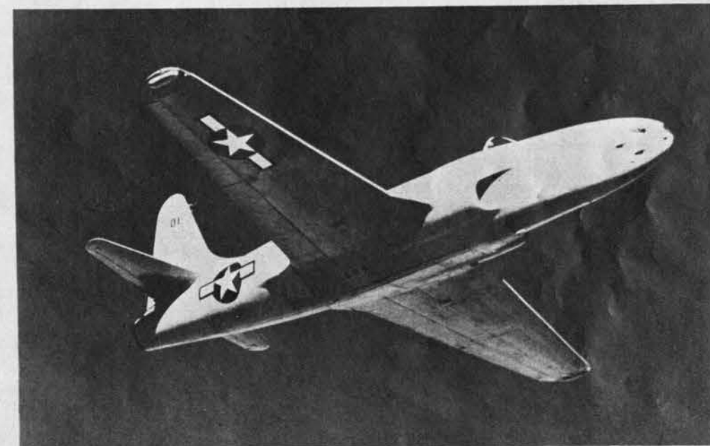
Shooting Star's wing has curved tips, even taper. Note wingtip shackles which support either bombs or fuel tanks. Vertical tail surface, which is rounded on top, curves sharply into fuselage.
